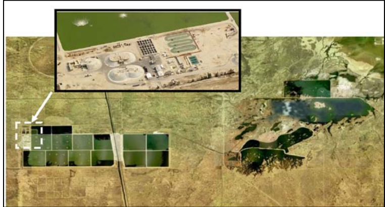
Photo 6 – Lancaster sewage treatment plant with treated effluent discharge to Piute Ponds
