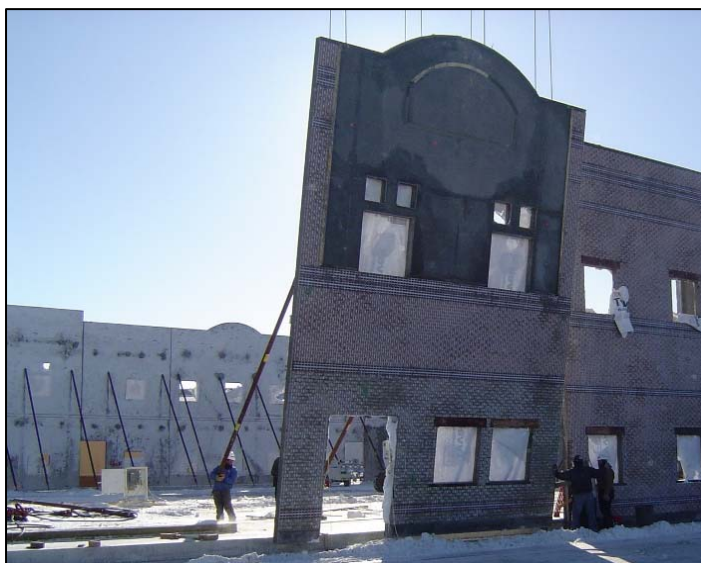
Photo 1 – “Tilt-up” building wall
